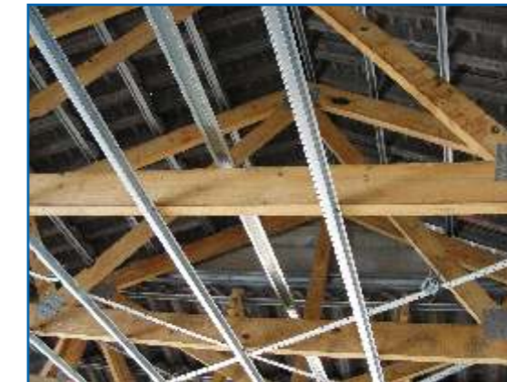
20mm Top-Hat ceiling branding installed on timber roof trusses with a concrete tile roof covering.
