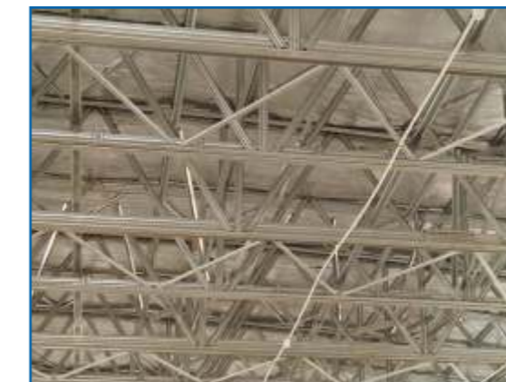
Top-Hat profiles used as bracing members in an Ultra-Span light gauge steel roof structure.
