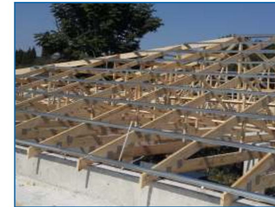
40mm Top-Hat profiles used as metal sheeting purlins on timber roof trusses.
